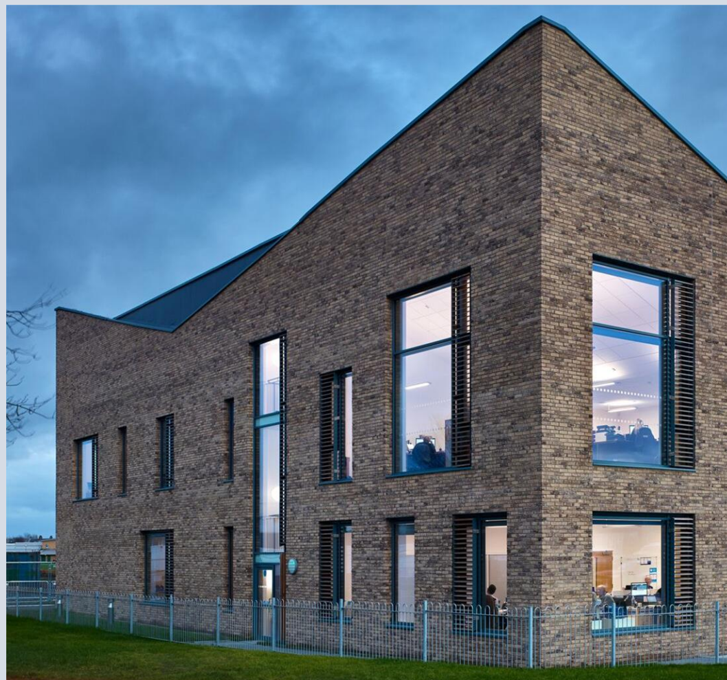
Redevelopment of derelict land at Quarry Road, Irvine.
