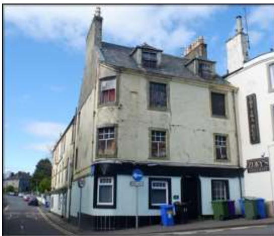
Category C Listed Building (at Risk)
